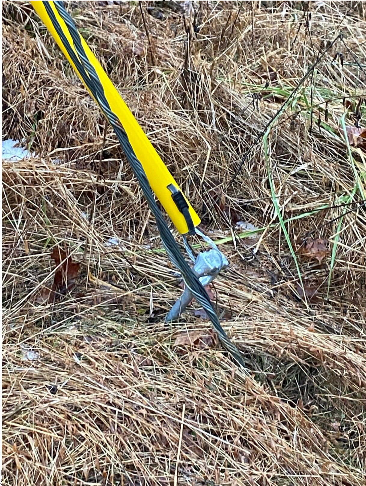
Figure 8 – Anchor is not installed in line with down guy. This allows for the potential of the anchor to be loosened back
